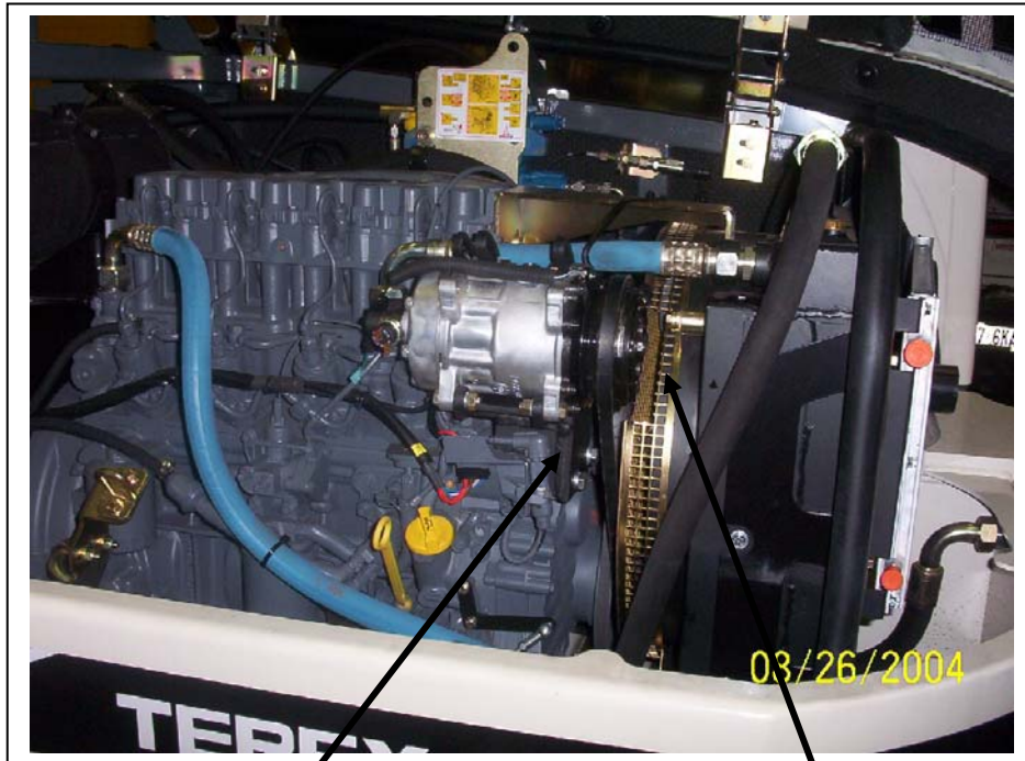
Main mount plate installed. Bolt it to the engine and the angled stiffener bracket. Use the supplied M10 bolts to attaché it to the engine and the 3/8" x 1 " bolt for the angled stiffener.
